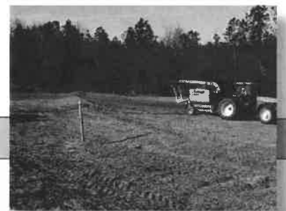
Reseeding the right-of-way
